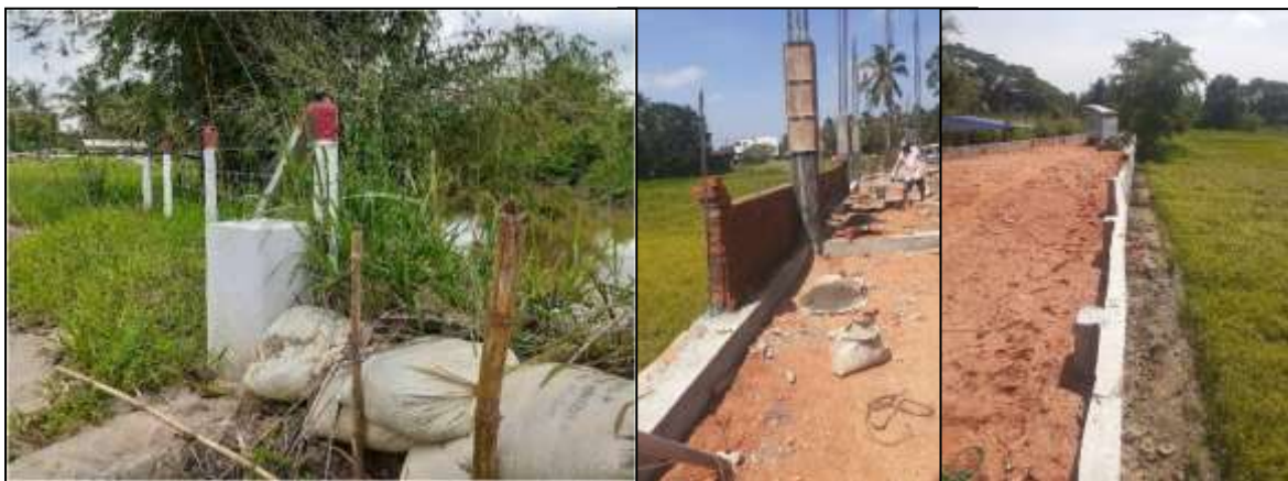
Figure No 3.2.2.: Pictures of development activities being carried out in eco - sensitive zones
